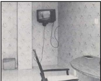
Television sets on elevated shelves must be securely restrained: the television bolted to the shelf or bracket, and the shelf properly anchored to the wall.
